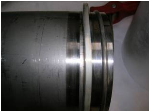
Figure 4. Deformed Welded Retaining Ring without Sleeves
